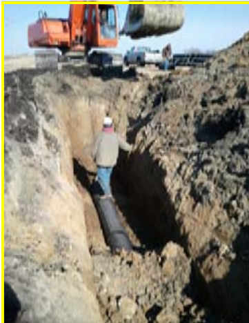
Above Left/Center: Digging in the main approximately 12 feet deep on Smeltzer #1
