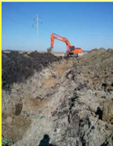
Above Left/Center: Digging in the main approximately 12 feet deep on Smeltzer #1
