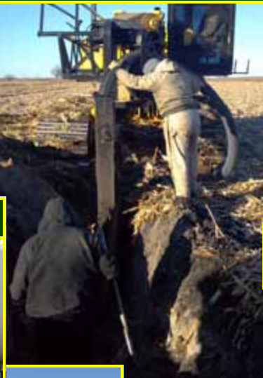
Above: Intalling tile on the Smeltzer #1 farm just north of the Nh3 plant.
