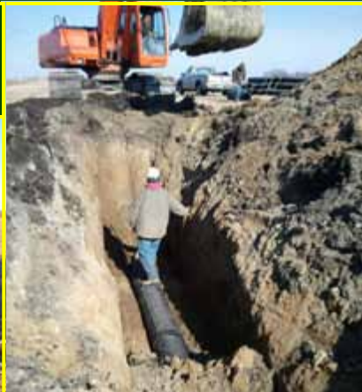
Above: Intalling tile on the Smeltzer #1 farm just north of the Nh3 plant.
